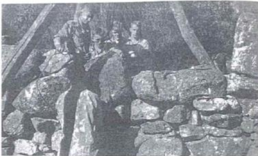
Lifting large rocks, using tripod and block and tackle, left to right: Geoff Goadby, Murray Rich, Tom Brown, Peter Reimann (photo Duncan McPhee)
